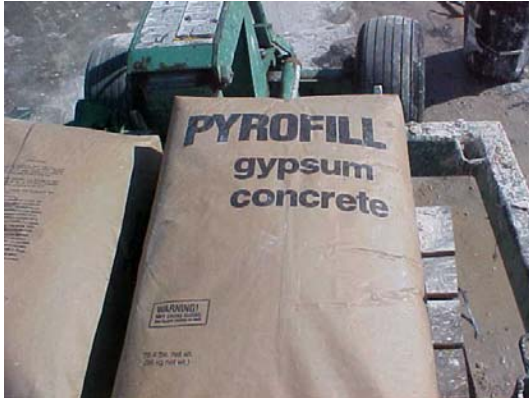
1. Bags of gypsum concrete
