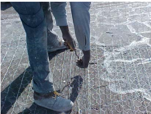
10. Installation of Ties to Connect Old Wire Mesh to New Wire Mesh Around Perimeter of Repair Area
