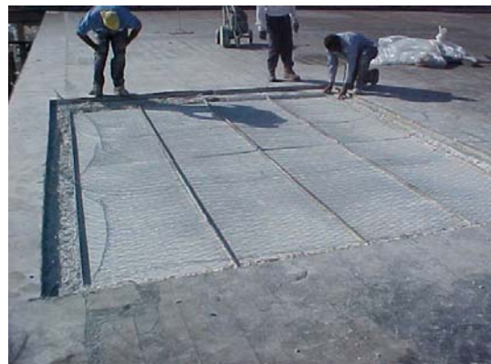
11. Completed Installation of New Wire Mesh
