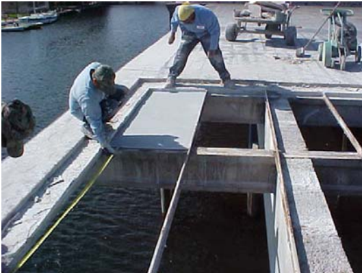
8. Installing New Form Board in Repair Area
