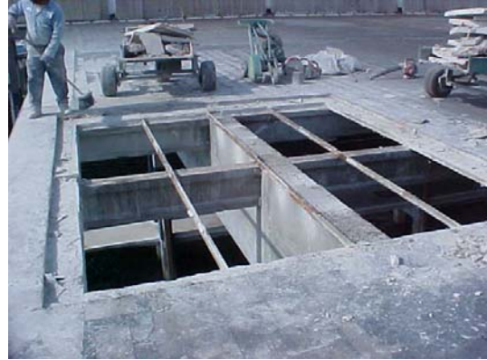
7. Section of Deck Removed Back to Structural Elements
