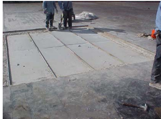
9. Complete Installation of New Form Board
